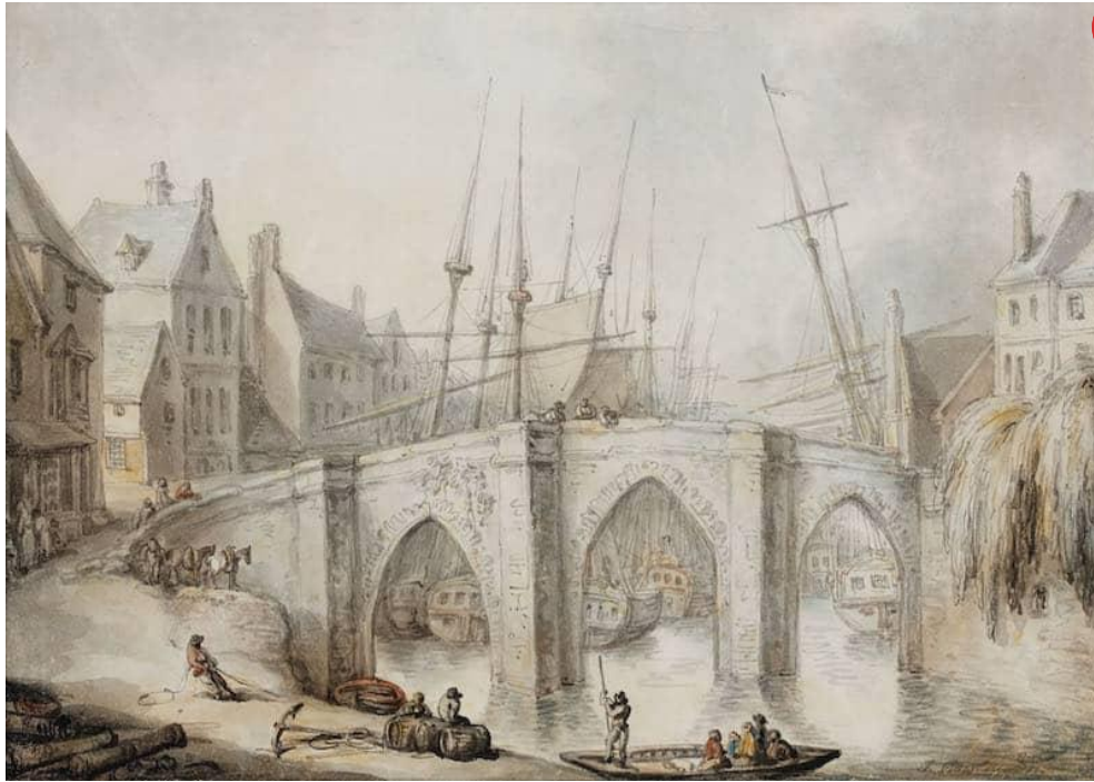
A bridge over a river in a town, with shipping moored
