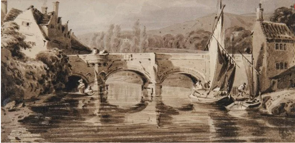
Bishop's Bridge, Norwich, from the south
